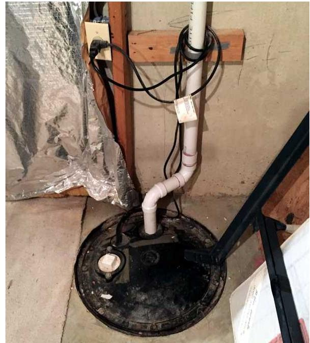
*Typical sump pump installation, with submersible pump, bypass float switch and white outlet pipe. Note the sealed crock cover with white inspection port plug.*
