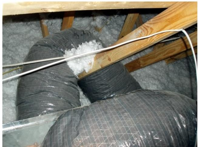
The bend radius at the center line of ducts shall be equal to or greater than one duct diameter. Sharper bends increase pressure drop significantly and reduce airflow.
