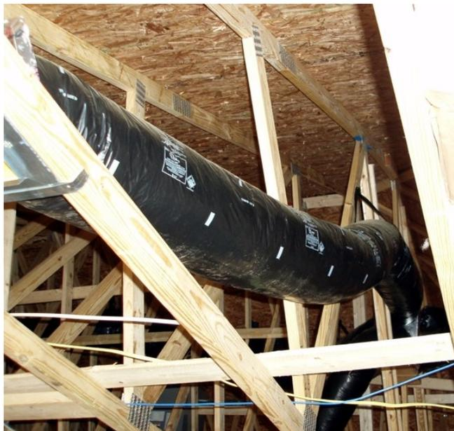
*Incorrect: Duct supports are greater than 4' apart, leading to excessive sag.*
