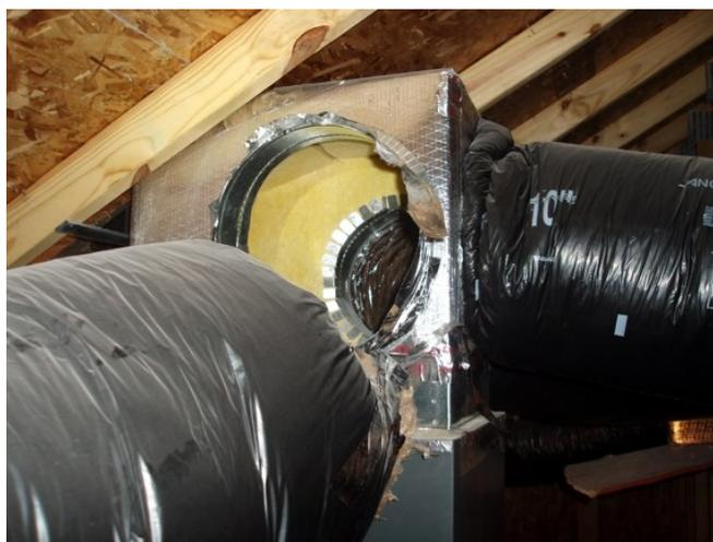
*Incorrect: Lack of flexible duct support can lead to the duct separating from the manifold, leading to energy loss and ineffective heating and cooling.*
