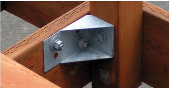
*Example of a steel connector that prevents railing post failures.*
