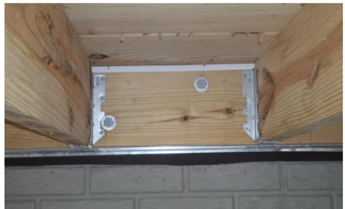
*What a proper deck attachment looks like: staggered bolts, proper joist hangers, uncorroded fasteners, bituminous and cap flashing. We rarely see them done this well.*
