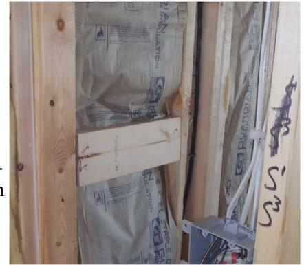
The other common trouble spot is around electrical boxes. Again, the insulation should be trimmed to fit around the box, and the space directly behind the box insulated with a piece of rigid or sprayed foam.
