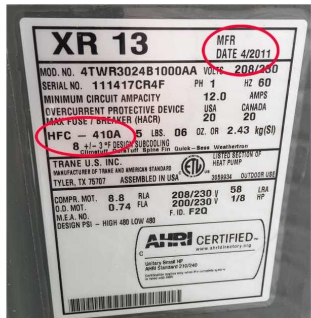
*This 13 SEER unit was manufactured in 2011 and uses the newer R-410A refrigerant. The seller claimed the system had been replaced in 2014; it's possible that a "new old stock" unit was installed.*
